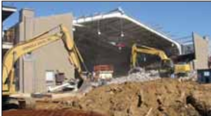
Crews removed the back wall of the Fieldhouse during the renovation.
