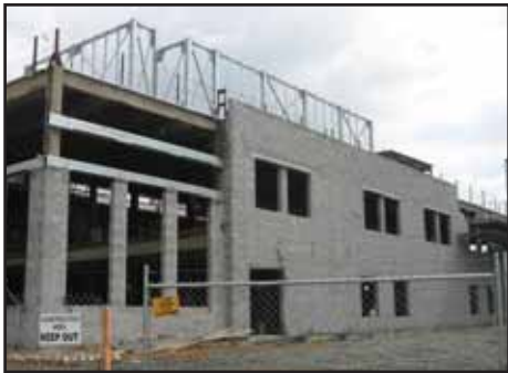
Construction of the Basketball Center has progressed quickly.
