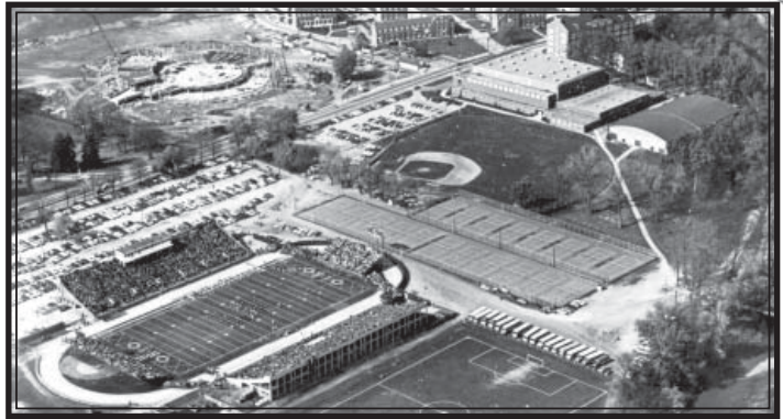
A view of the athletics mall in 1967. Construction of The Convo was in its beginning stages.
