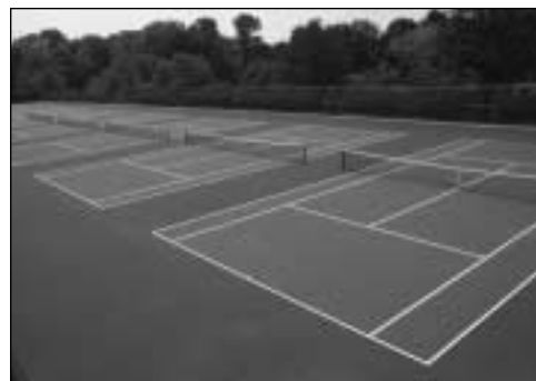
West Campus Tennis Courts
