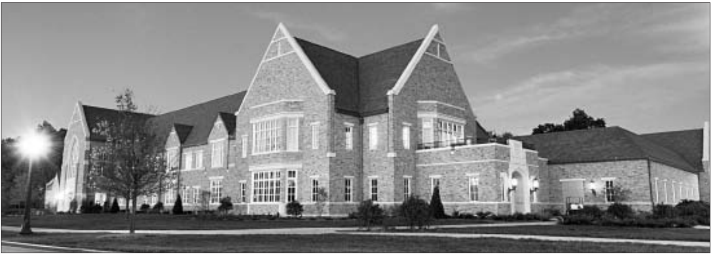
The Guglielmino Center, opened in August of 2005, is the home of the Hagggar Fitness Center – Notre Dame’s strength and conditioning and weight room equipment area for all 800 Irish student-athletes.
