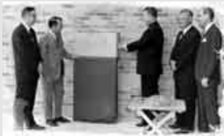
Father Joyce (third from right) is shown laying the cornerstone of the Athletics and Convocation Center in 1968, the building that now bears his name.
