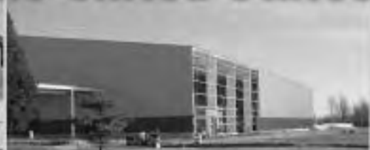
Brigade Sports Complex (Under Construction) Tennis
